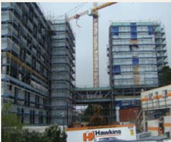
Design and construction of three student accommodation towers at Victoria University in Wellington.
